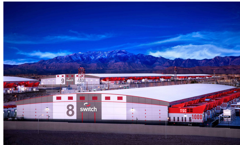
Photo courtesy of Switch
