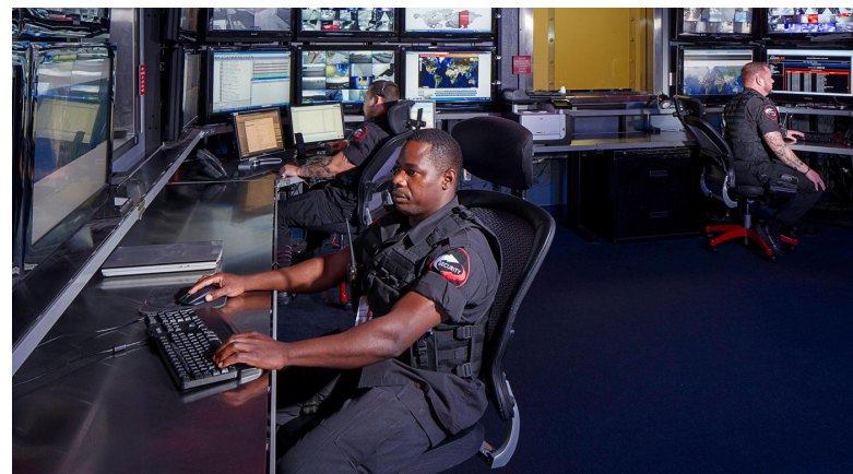
Photo courtesy of Switch
