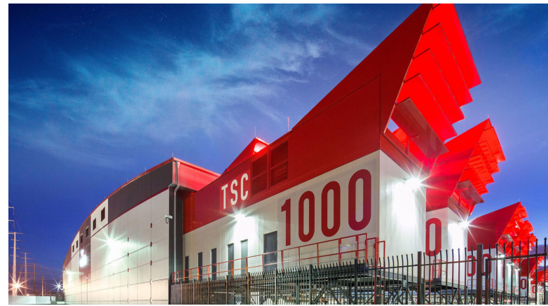
Photo courtesy of Switch
